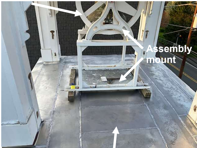
New aluminum roof on lower section
