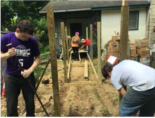
One team was building a handicapped ramp.
